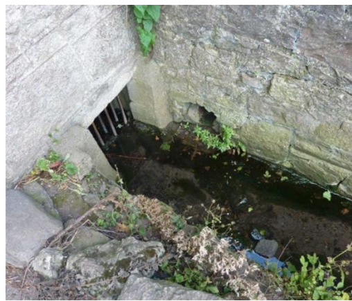
Photos of the grated wall opening for drainage at Locations B2 (left) and B1 (right)
